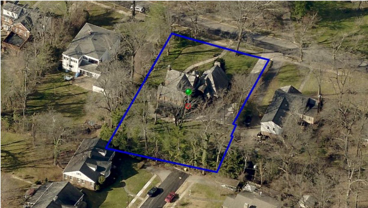
Exhibit 7: Aerial view east elevation 2020 Pictometry
